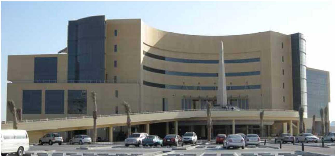
The newly opened Royal College of Surgeons in Ireland—Medical University of Bahrain
